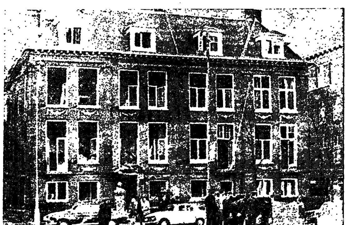
Heavily damaged Soviet trade delegation building in Amsterdam after explosion.
